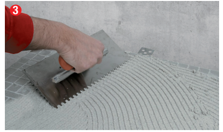
3 Laying the glue on the slab and wall
