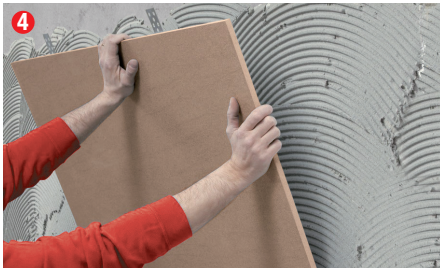
4 Install the slab to the wall with glue
