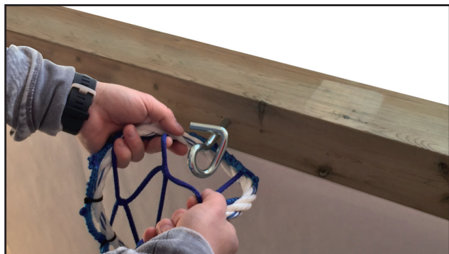
1) Standing in front of the hook, grab the net with both hands and place it under the hook opening
