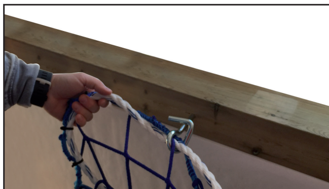
4) The network has entered into the hook. proceed to the next hook
