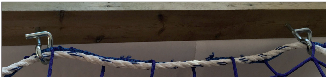
5) The network is entered correctly into the support hooks
