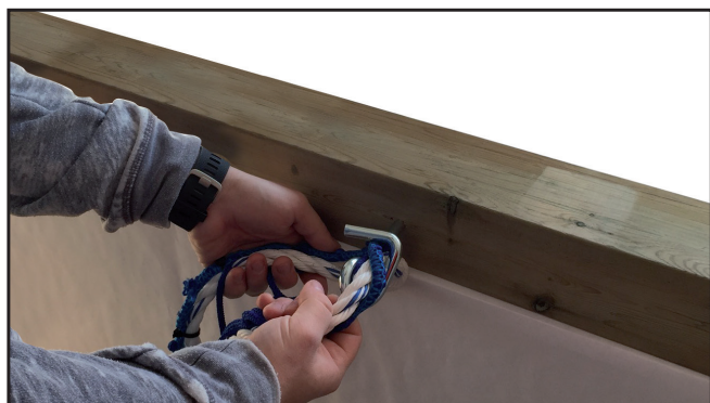
3) Hold the net with both hands pulling the ends to facilitate the move into the hook
